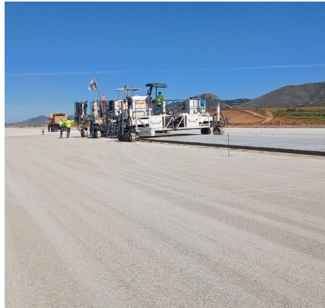
Runway Lean Concrete Paving
