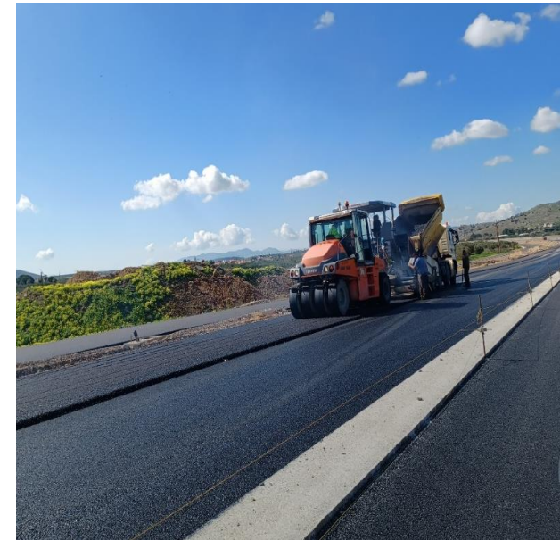
External Road Asphalt paving
