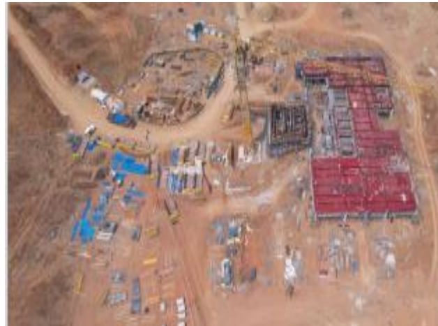
Air Traffic Control Tower
