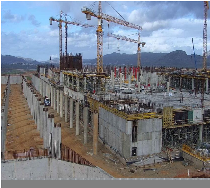
Terminal Building Structural Concreting works
